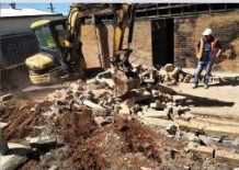
Rebuilding Start, Oct. 2018
